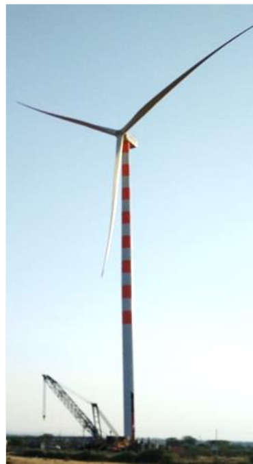
S120 – 120 STT (Jan '19) Smart Tubular Tower
