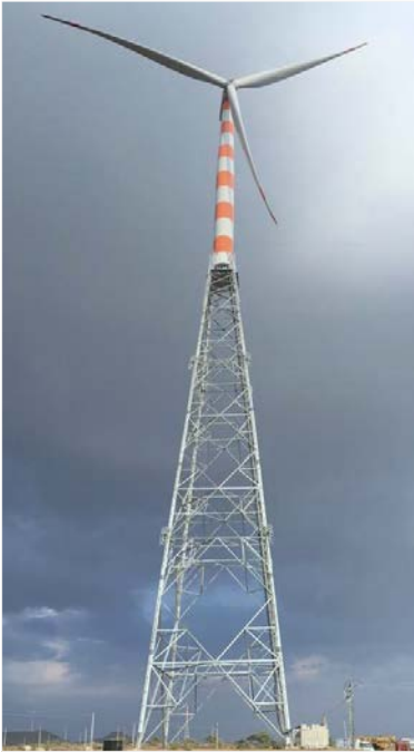
S120 – 140 HLT (Dec '18) Hybrid Lattice Tower
